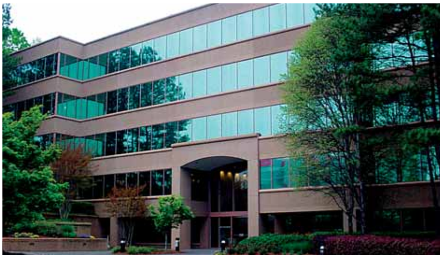
■ Melaver's Crestwood Building, Atlanta, recently earned LEED-EB certification. >> Photo by Brad Feinknopf/Feinknopf Photography.
